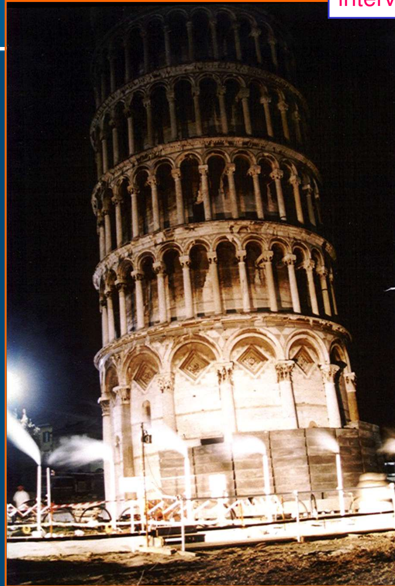
Freezing in operation with exhausted nitrogen
